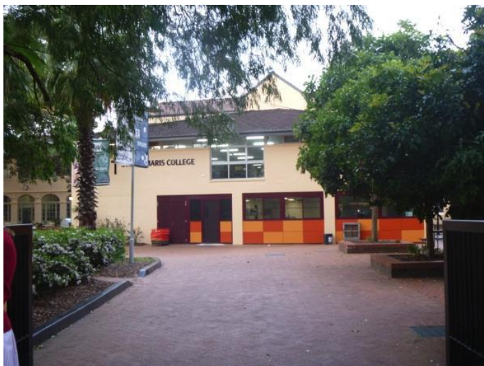
SCHOOL CANTEEN BUILDING
