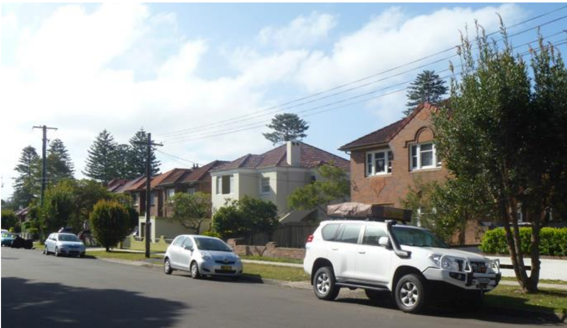
HERITAGE LISTED TWO STOREY RESIDENTIAL FLAT BUILDINGS ALONG THE NORTHERN SIDE OF EUROBIN AVENUE
