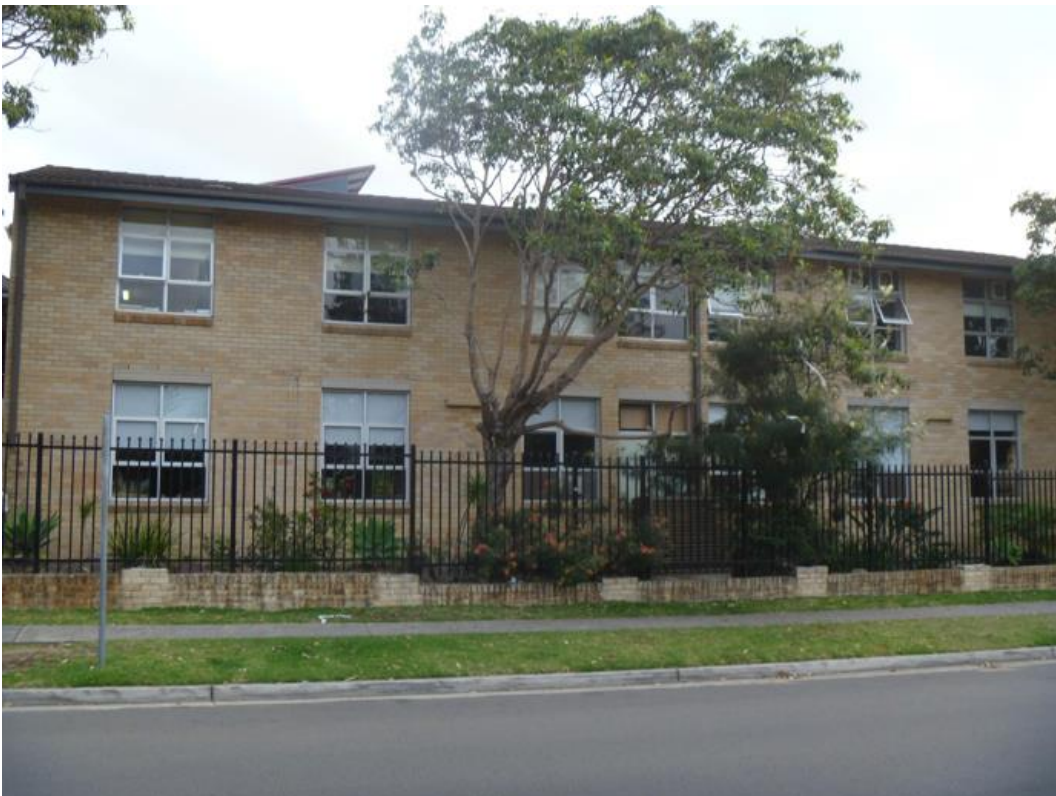
'E' BLOCK WITH FRONTAGE TO EUROBIN AVENUE (TO BE DEMOLISHED)
