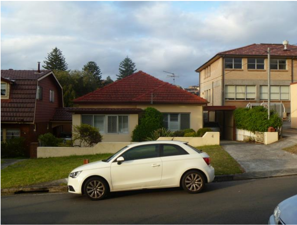
ADJOINING SINGLE STOREY DWELLING HOUSE (4 ILUKA AVENUE) TO THE NORTH-WEST OF THE LOCATION OF THE NEW SCIENCE BUILDING
