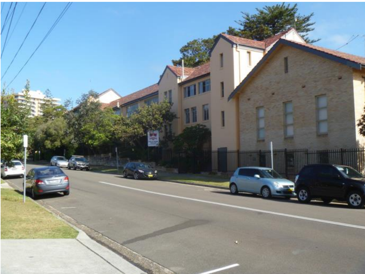
SCHOOL HALL BUILDING AND 'E' BLOCK WITH FRONTAGE TO EUROBIN AVENUE
