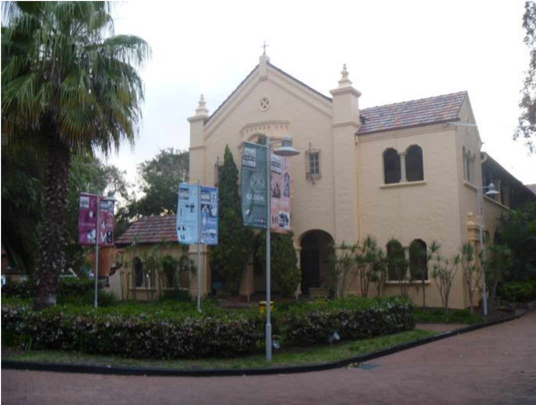
INTERNAL VIEW OF CONVENT
